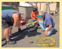
welder was used to weld the new pipes to the existing poles and new beams over the frame.
