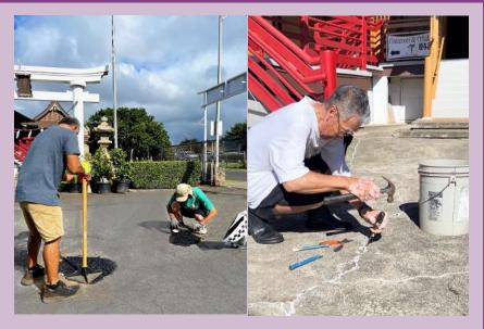
At some point in time, all parking lots require pothole repair. Potholes, alligator cracking, water from rain or inadequate drainage can seep into the asphalt, causing it to crack and split
