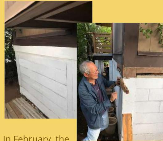
In February, the wooden trim on the exterior wall of the shrine was removed and repaired due to termite damage.
