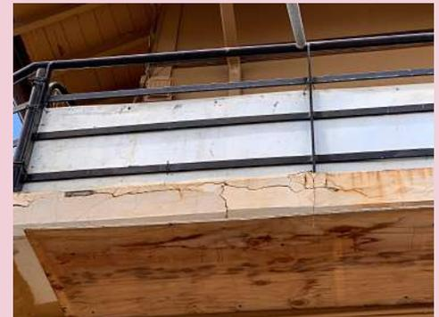
Presently, the spalling damage is seemingly about 1/3 of the thickness of the concrete.
