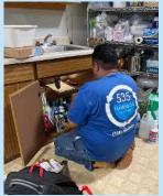
The meeting room's faucet began leaking at the base. The worn out valve took the plumber over an hour to remove as it was fused to the pipe. It was the first time the faucet was replaced since it was first installed in 1980.
