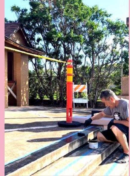
A non-skid paint was applied to the steps to increase traction and slip resistance.
